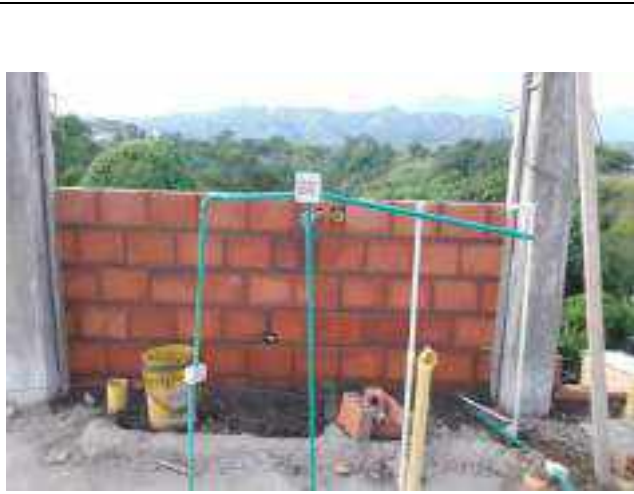
Instalacion tuberia electrica torre B
