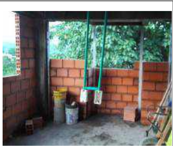
Instalacion tuberia electrica torre a
